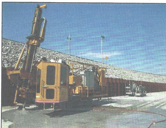
FIGURE 12. Crawler drill rig with Water-Powered Down-the-Hole (WDTH) Hammer (Source: ACT, Ltd.)
