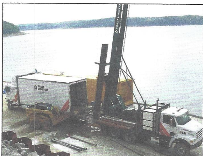
FIGURE 11: Truck-mounted Sonic Drill (Source: ACT, Ltd)
